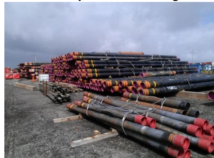
Current Lay Down and Storage base
