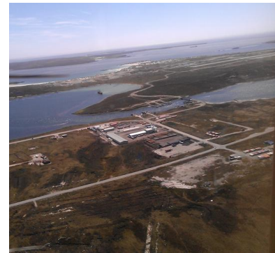
New O&G Lay-Down Areas
