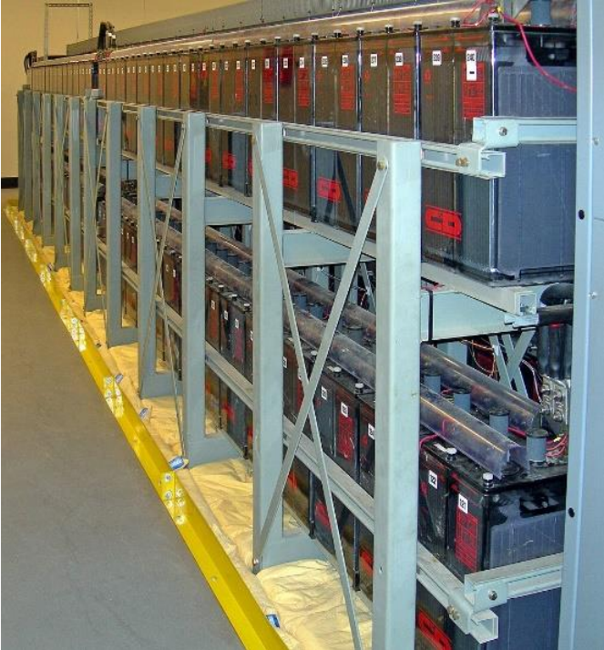
Battery storage is a widely used form of energy storage for renewable systems and anticipated to be the initial form of energy storage for Stanley. Photo credit: Wikipedia.
