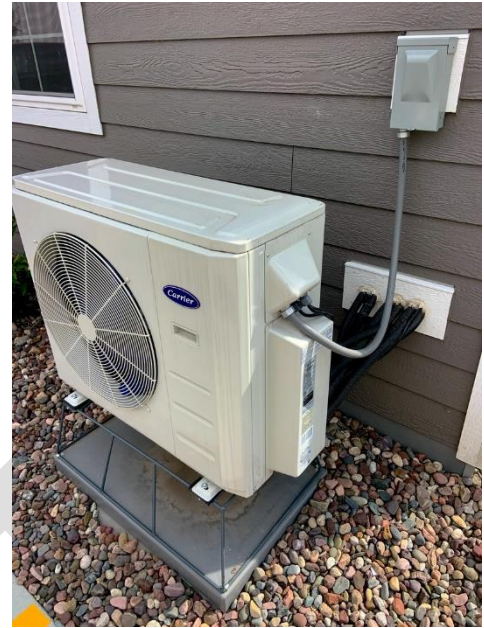
Heatpumps are a sustainable heating option, but work best where buildings have first been properly insulated. Photo credit: Wikipedia.
