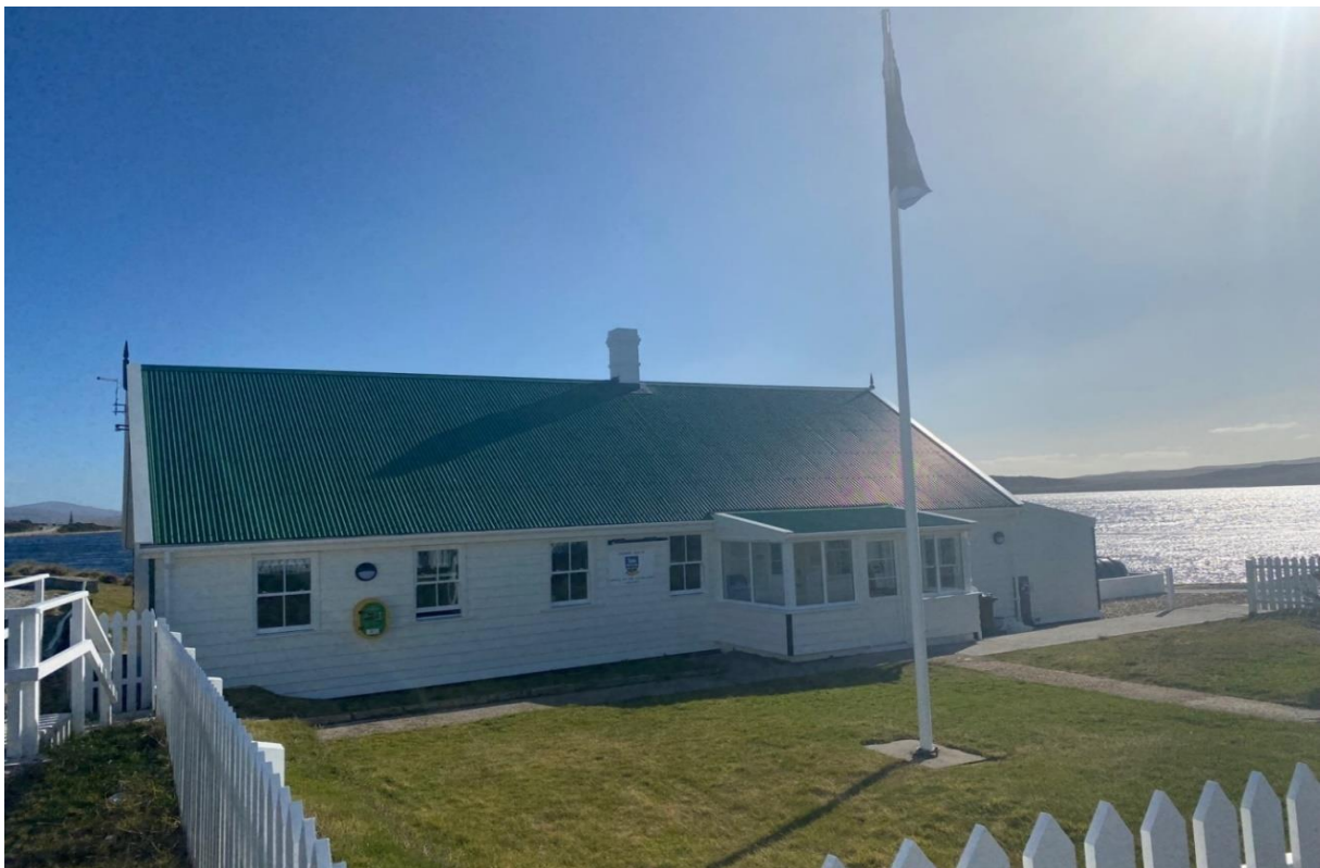
12. “Gilbert House” courtesy of the Falkland Islands Government Home to the either elected members of the Legislative Assembly, Gilbert House was built in the 1850s. It has had many uses over the decades including as a hospital, headquarters for the Falkland Islands Defence Force and the original home of the government archives.
