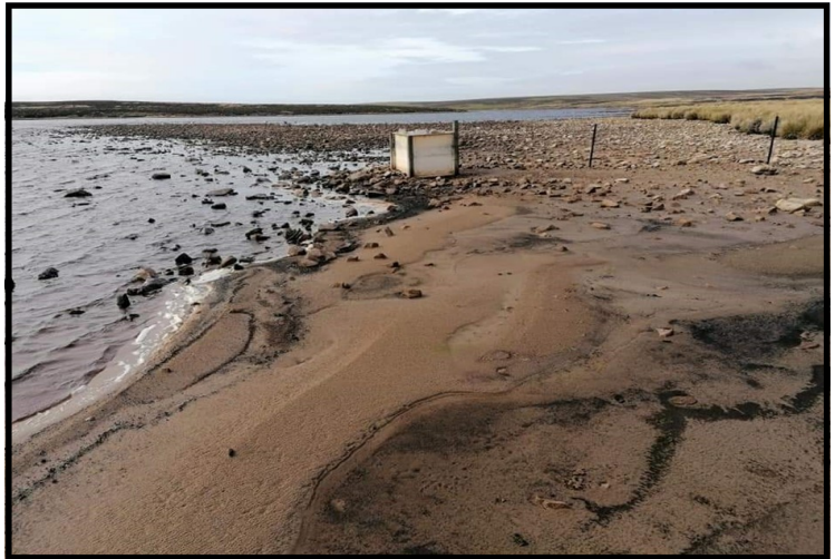
Low water level in ponds: high and dry gabions and fences are no longer effective stock barriers – photo credit Ben
